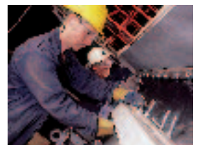
Expansion joint installation
